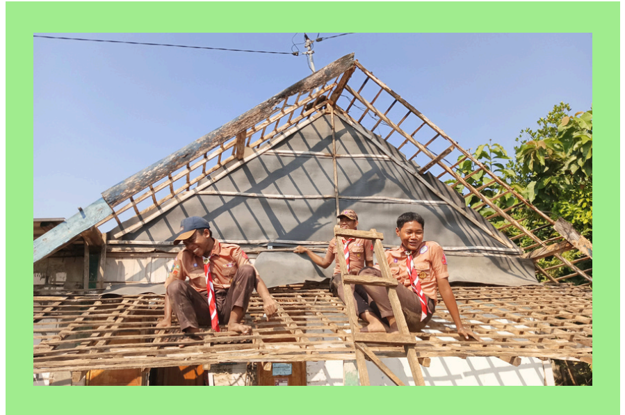
Scouts doing roofing works on one of the houses.
